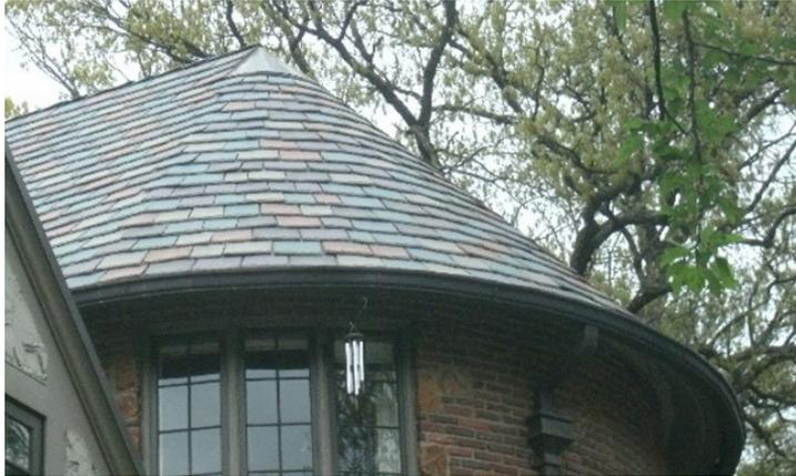
be effectively coverable with the Niagara Slate or Shake profile. Because of the ribbed design of the tiles, it is not recommended to cut the exposed portion of the tile to the roof angle as described in the Majestic/Empire Slate and Seneca/Empire Shake instructions. Instead, the angle cut would be from the top of the tile, ending at the side of the tile even with the nail location.
