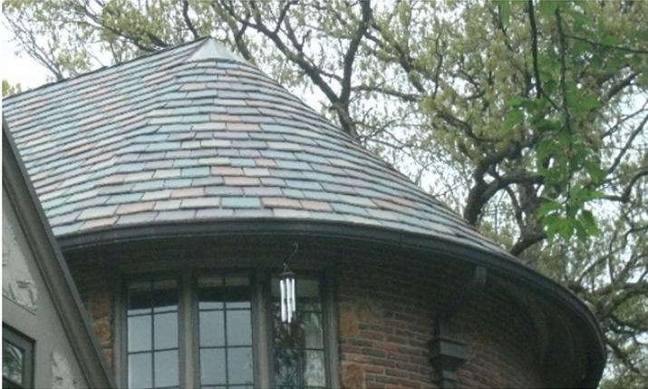
Because of the ribbed design of the tiles, it is not recommended to cut the exposed portion of the tile to the roof angle as described in the Majestic/Empire Slate and Seneca/Empire Shake instructions. Instead, the angle cut would be from the top of the tile, ending at the side of the tile even with the nail location. **See Figure 1.**
